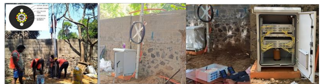
Aerial Deployment: Pole Installation, Cable Pulling & Termination & Splicing
