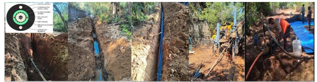
UG Deployment: Digging, Trenching and Ducting, HDD, Cable Blowing
