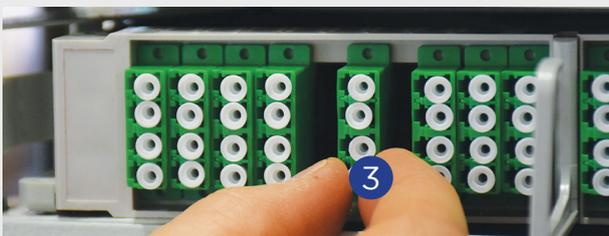
3. The space is useful for moving every single set of pigtail connections
