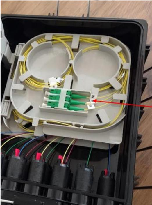
When making a spliced network connection, cut splitter input tails here. Then remove tails from middle tray.
