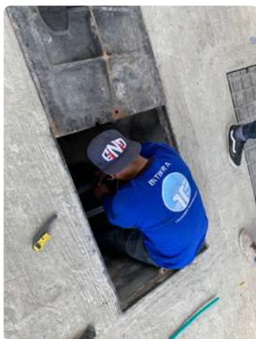
Manhole at Midsection
