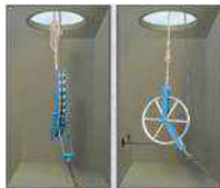
Sheaves and quadrant block in manhole
