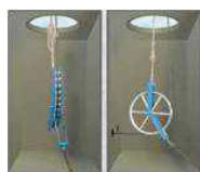
Sheaves and quadrant block in manhole
