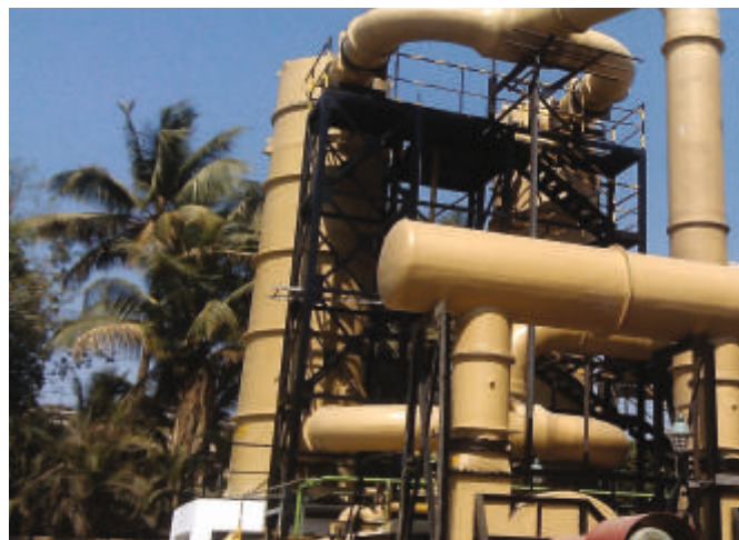
Scrubbers to Remove Harmful Pollutants from Gases at Waluj
