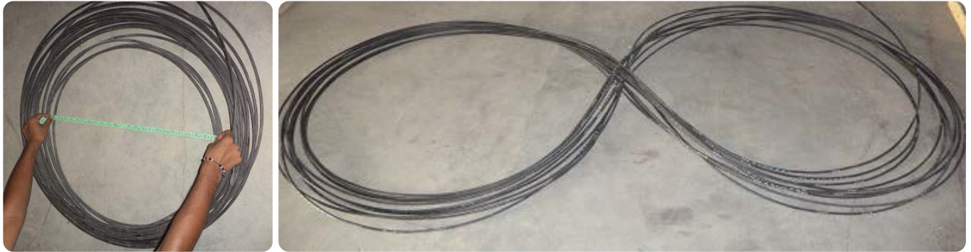
Figure 5 - Cable coiling in manhole or hand-hole and intermediate pulling/blowing
