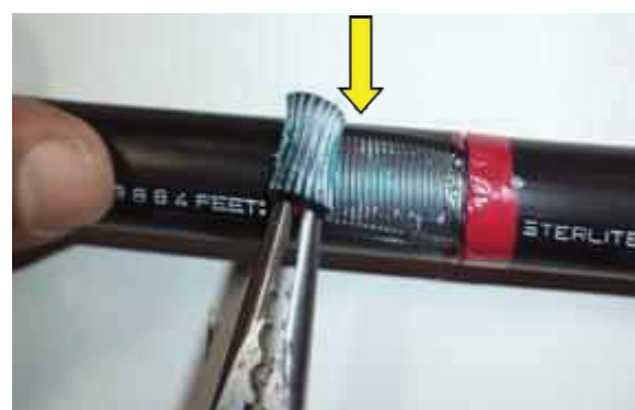
Figure 6- Removal of outer jacket by nose pillers at the 15 cm window
