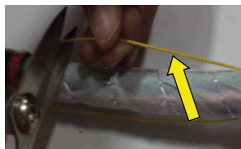
Figure 11- Cut the rip cord thread over the water blocking tape/ polyester tape using scissor
