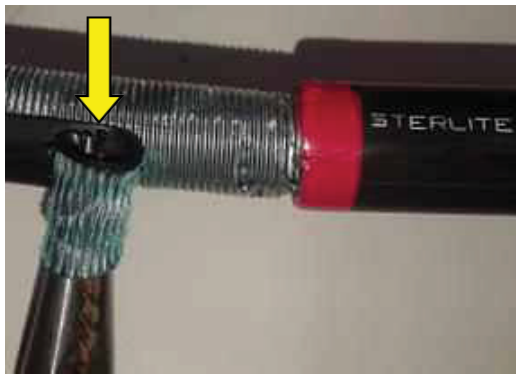
Figure 7- Removal of outer jacket by nose piller at the 15 cm window
