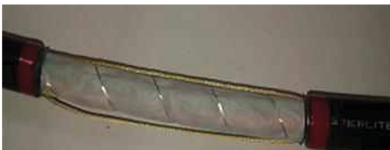
Figure 10- Exposed rip cords at the 15cm mid-span window
