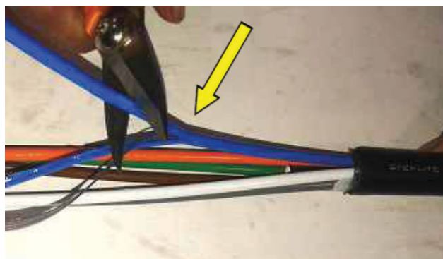
Figure 19- Removal of tube covering by scissor
