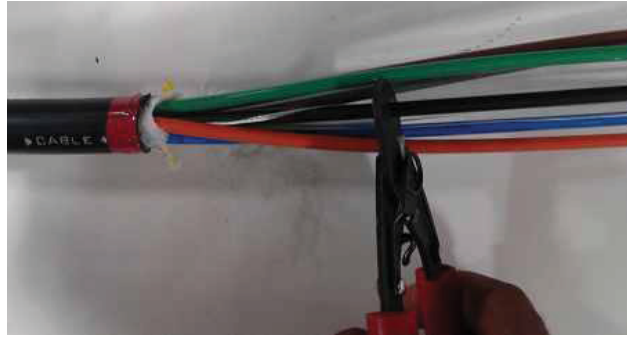
Figure 17- Removal of the center strength member using small cutter
