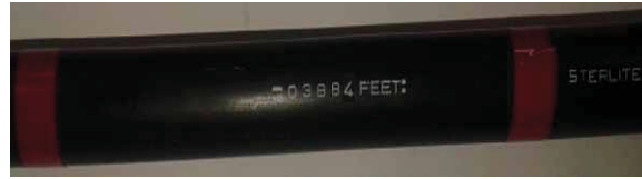
Figure 2- Markers for mid-span access
