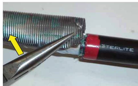
Figure 9- Removal of metallic tape by nose pliers for 15cm window cut portion
