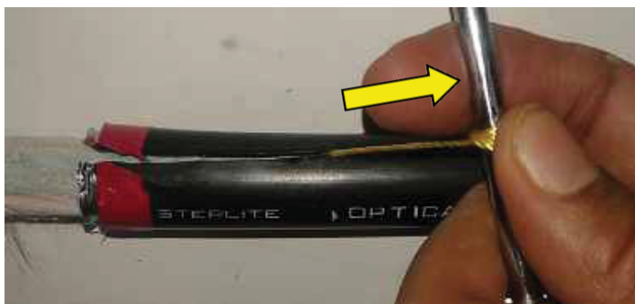
Figure 12- Slitting of cable jacket by using rip cord
