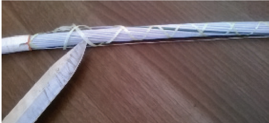
Figure 11 Cut the binder yarns over the bundled loose tubes.
