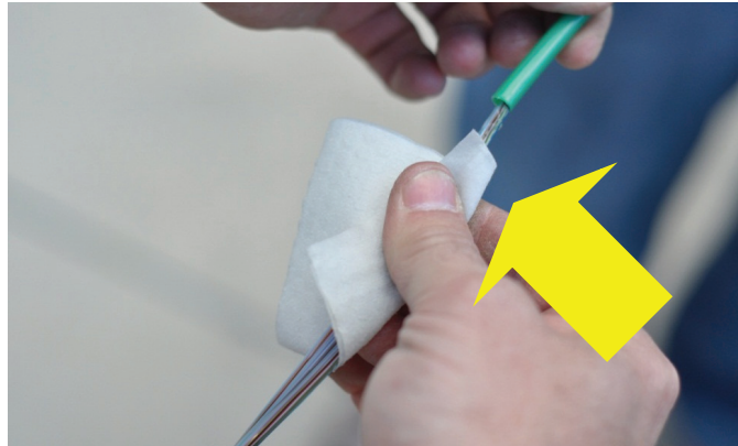
Figure 18 Wipe the water blocking gel from the fibers.
