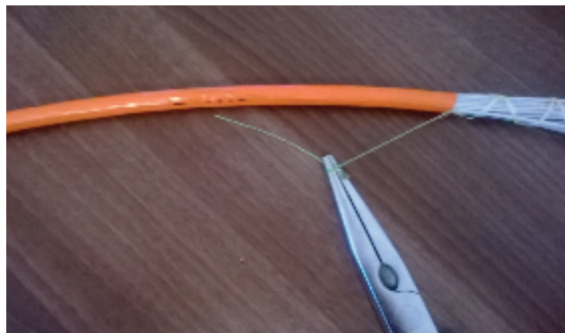
Figure 24 Slitting of cable jacket using rip-cord.
