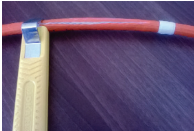
Figure 21 Cable sheath being scored with sheath cutting and slitting tool at the 15 cm window near the center of mid-span access window.
