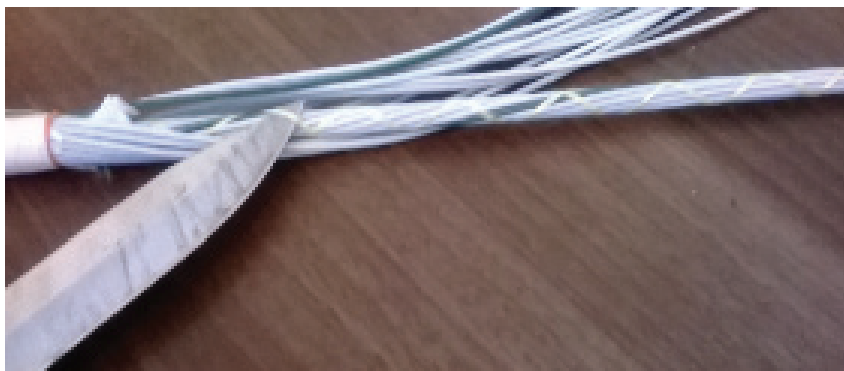
Figure 13 Remove the binder yarns which bundles tubes on the inner cable core (in case of dual layer microcable design).
