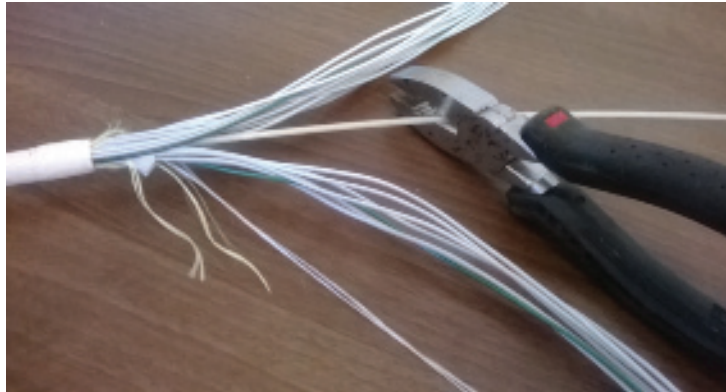
Figure 29 Removal of the center strength member using small cable cutter.
