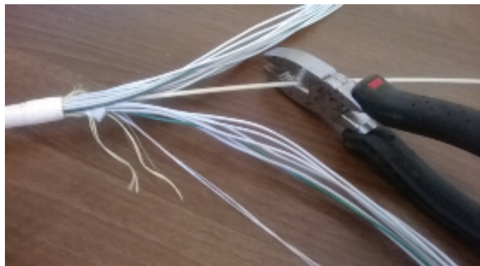
Figure 15 Trim the cable strength members to mate properly with the splice closure.
