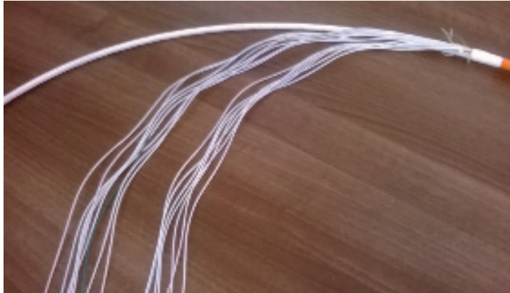
Figure 14 Unwind the loose buffer tubes in the cable core from around the CSM.
