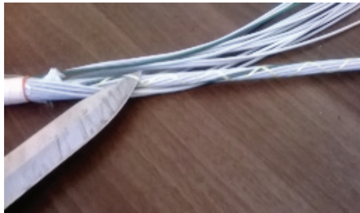
Figure 27 Remove the binder yarns which bundles tubes in the inner cable core.
