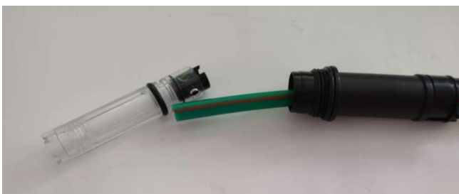
Pass the 7mm duct through the outer housing as shown. The end of the duct must be rounded off to make it easier for the next part of the install.
