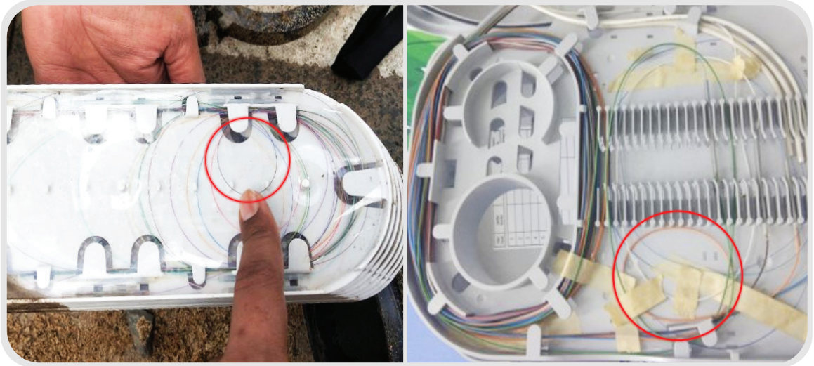
Figure. 1 Tight fibre bends in a splice tray
