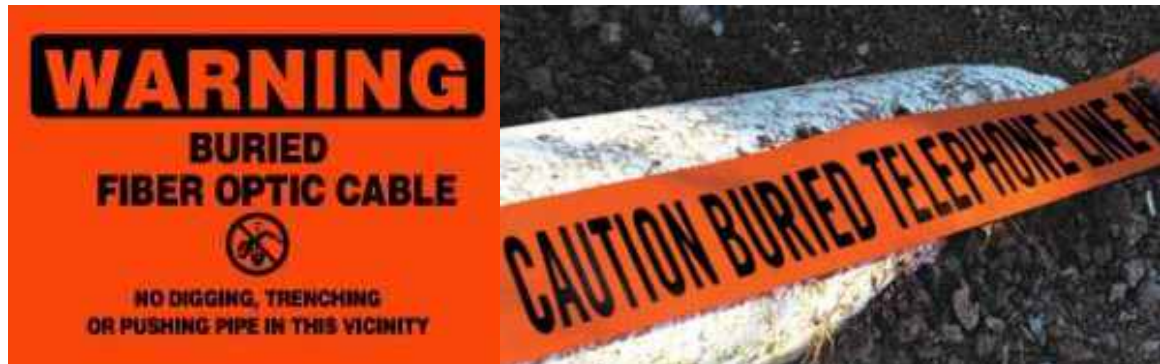
Figure 2– Fiber Optic Marking Tape and Warning Sign
